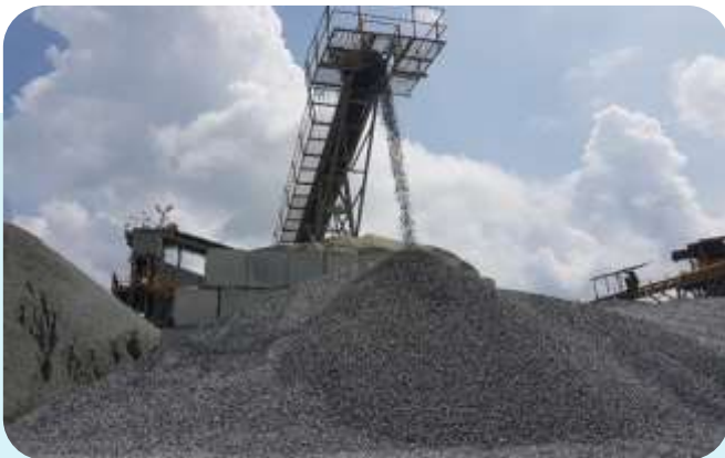
Construction & Demolition waste recycling
