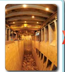
The Plant has four high capacity rotary bulky waste crushers integrated in the waste reception hall so that waste trucks are able to discharge their loads directly into the crushers. A bulky waste pit, which is a temporary storage facility, allows peak intake of bulky waste to be stored and crushed during off-peak hours.
