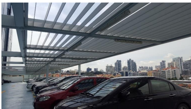
Figure 102: A Basic Brise Soleil As Shading Device For Vehicles At The Outdoor Carpark Of CENTRAL Mall In Singapore. (Courtesy: Patricia Collera)
