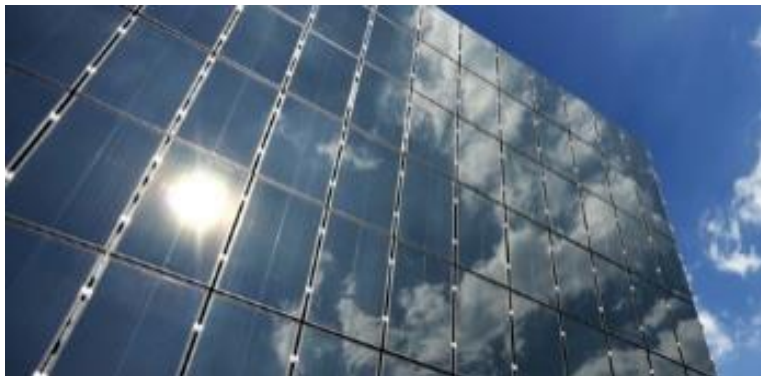
Figure 143: BIPV Façade With CIGS Film Solar Modules (Courtesy: Mansz-AG, www.manz.com )
