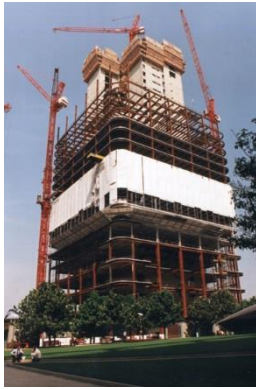
Figures 28 And 29 Unitised System Under Erection And Completion (Courtesy: Fosters + Partners Pte Ltd (Fig 28) and Pixabay.com (Fig 29))
