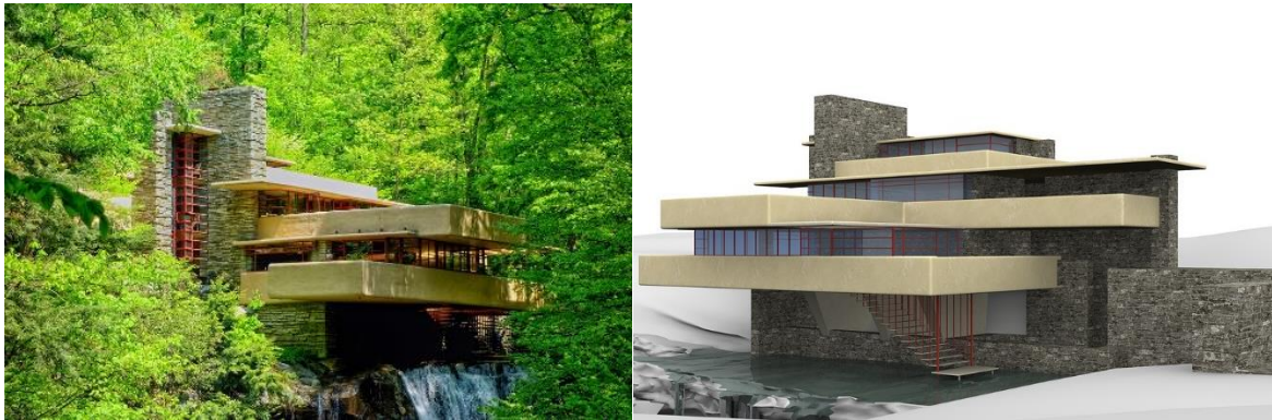
Figure 8 External View Cantilever RC Decks (Courtesy: Pixabay.com)
