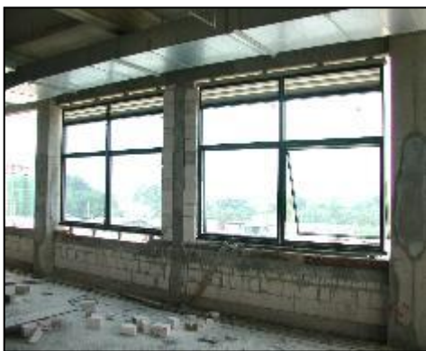
Figure 34 Stick System Under Installation
