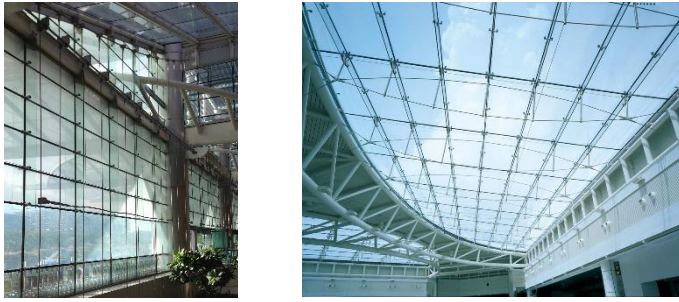
Figures 62 And 63: Cable-Net System (Detail And General View)
