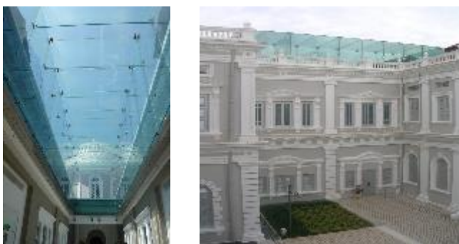
Figures 64 And 65: Glass Used In More Structural Applications As Vertical Supports And As Fin Stabilizers
