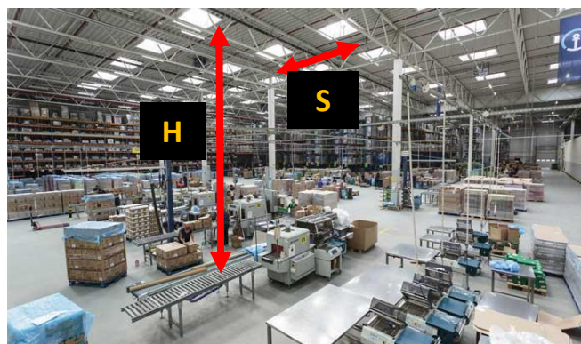
Figure 266: Spacing To Height Ratio Of Luminaires (Image Credit: Philips Lighting)
