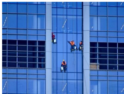
Figure 113 Use Of “Spider Man” For Maintenance
