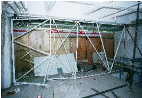
Figures 152 Steel Frame
