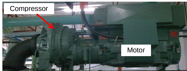
Figure 1.17 Photograph of an open-type compressor system
