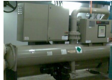
Figure 3.7 Water-cooled chiller
