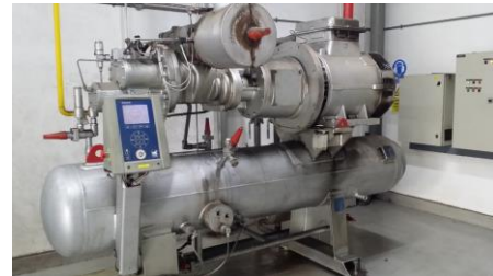
Figure 3.13 Screw type refrigeration
