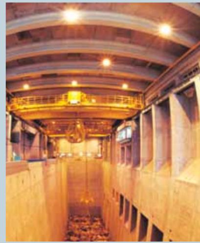
**3** The Plant has four high capacity rotary bulky waste crushers integrated in the refuse reception hall so that refuse trucks are able to discharge their loads directly into the crushers. A bulky waste pit, which is a temporary storage facility, allows peak intake of bulky waste to be stored and crushed during off-peak hours.
